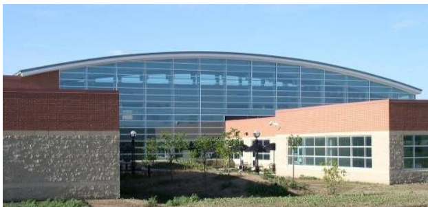
Buildings which are carefully articulated and massed to promote distinctive character and community identity are encouraged, as illustrated above.
